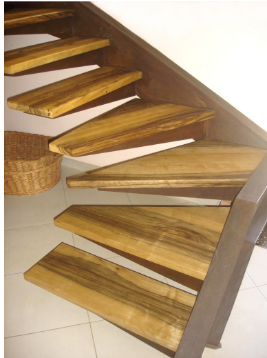
Half turning suspended staircase (dark colored figured afara) - Saint-Gély-du-Fesc (France)
