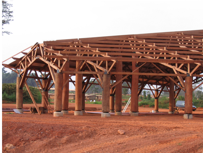
Triangular structure in Kosipo and posts in Tali – By J.Y. Riaux - Mindourou (Cameroon).
