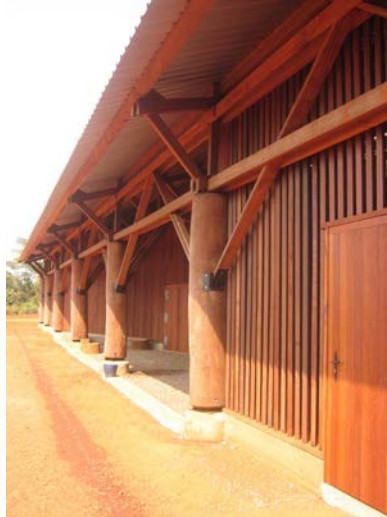
Door in Moabi, posts in Tali, framework in Kosipo, vertical thin timber cladding in Mukulungu – J.Y. Riaux, Mindourou (Cameroon).
