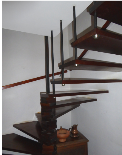
Half turning suspended staircase - Argelès/Mer (France)
