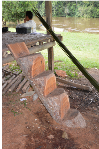
Staircase in Carapa for the Yawapa carbet (traditional gazebo-like structure) – Designed by Laurent Pilaoukou (French Guiana).
